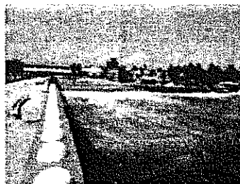
Plate 7. Pier at Valathura, Kerala
